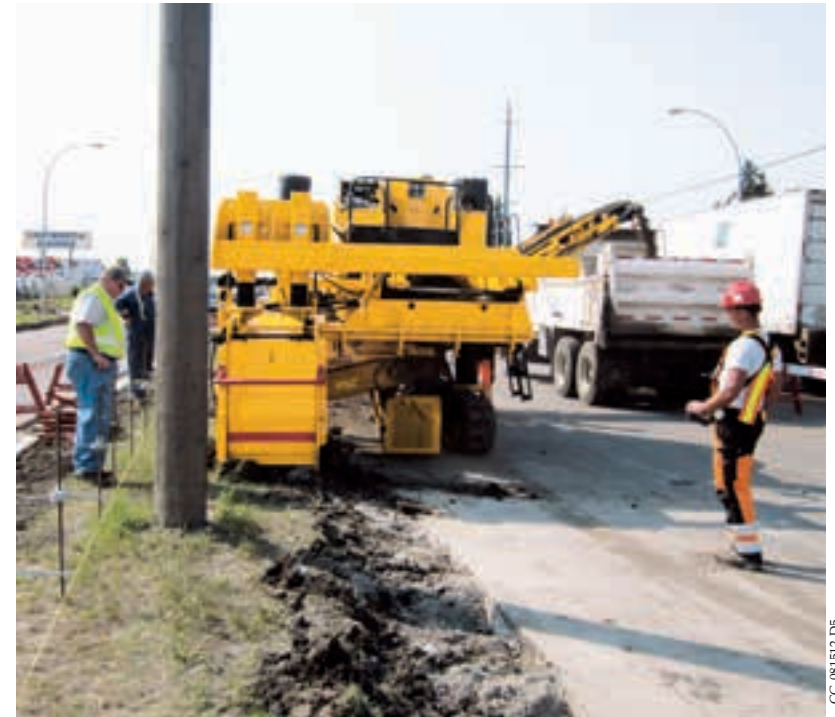
The 30 inch (762 mm) wide trimmerhead cuts 19 inches (483 mm) below grade on its first project.
