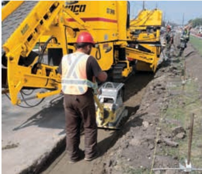
The blade on the trimmerhead was used to level the CTB material for final grade.
