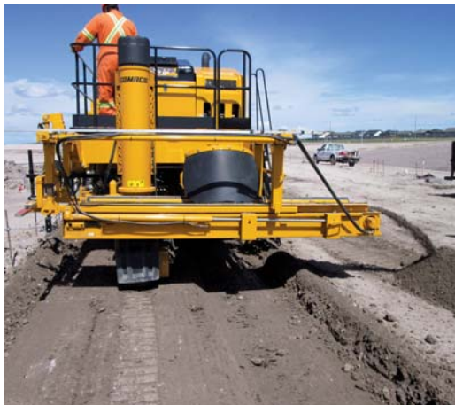
It is capable of trimming flat or monolithic sidewalk profiles up to 11 feet (3.4 m) wide.
