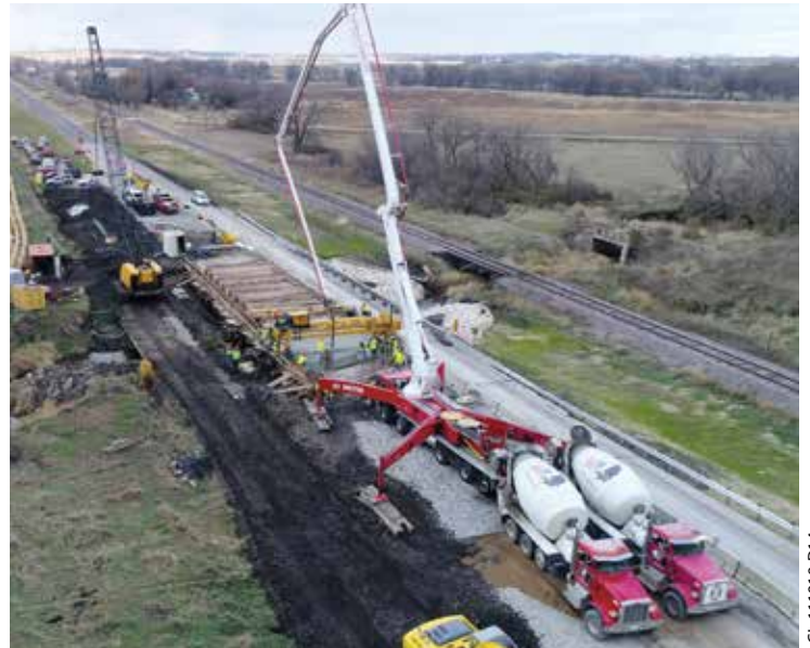
Two ready-mix trucks feed a concrete pump providing the C-450 and high-production screed with a constant supply of concrete to finish this 21 inch (533 mm) deep bridge project.
