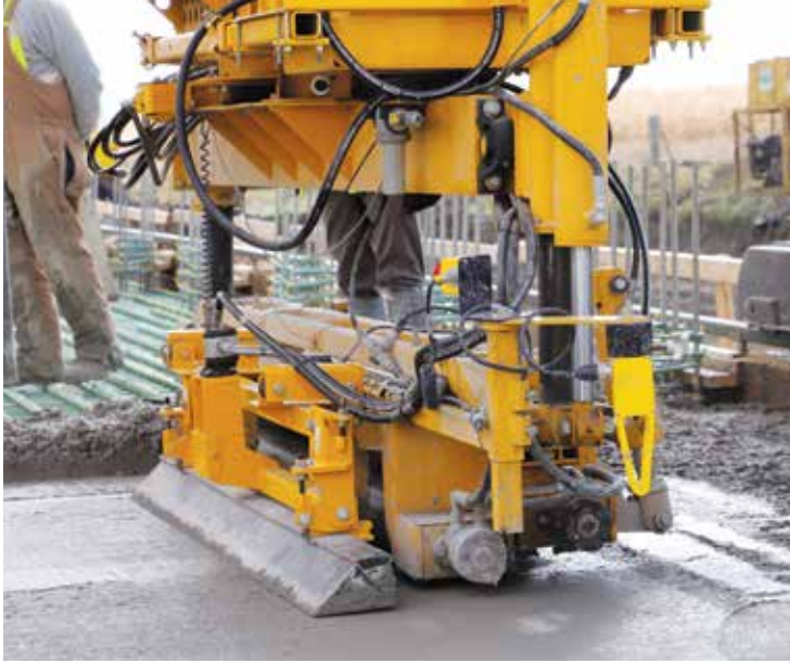
The revolutionary high-production screed has an auger, finishing cylinder, and trailing screed in series to finish the concrete in one pass.
