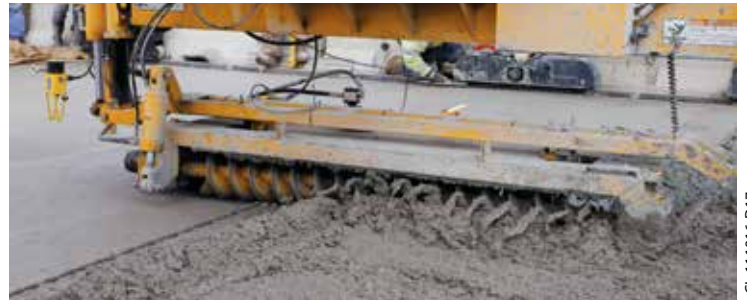
The 5.7 foot (1.74 m) long auger can advance as much as four feet (1.22 m) in a single pass.
